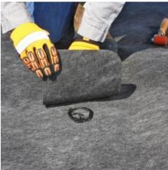
5) Center the patch over the hole or puncture and press down to spread the sealant.
