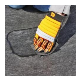
8) After the sealant has set (1 to 4 hrs), test the patch with the vacuum box for leaks. Fix any leaks with additional sealant or, if necessary, with a larger covering patch.
